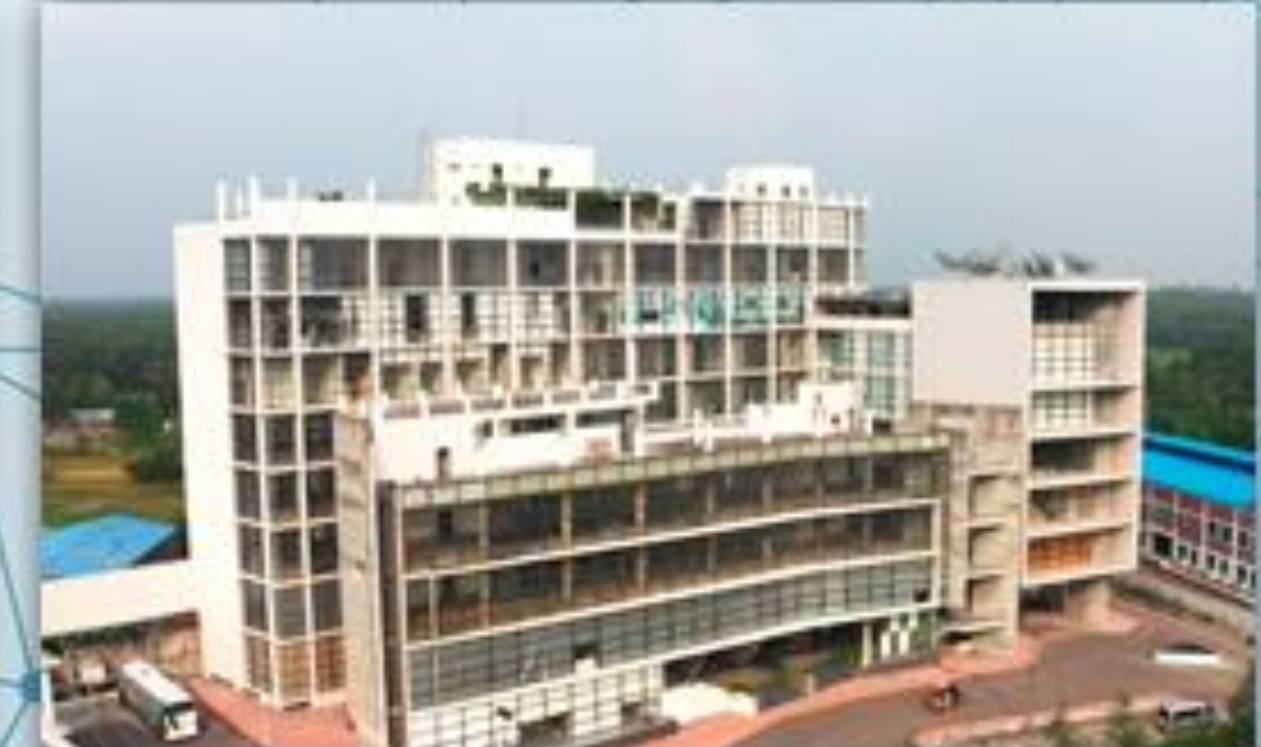
Solaris Building, Kaliakoir (1000+ Employment)
