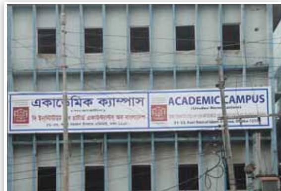
Renovation of the Bulding to start soon
